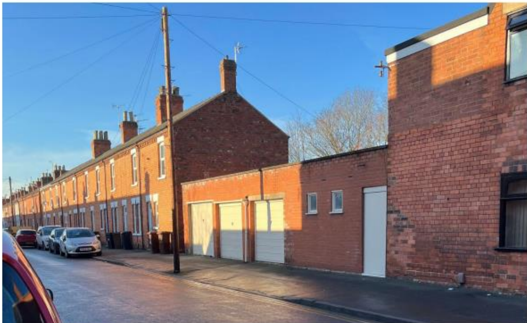
View 2 looking west towards the building, along Henley Street illustrating the poor elevational treatment and scale of the existing storage wing.
